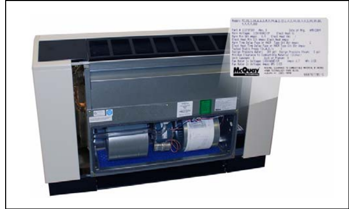
Figure 3: Data Plate Location
